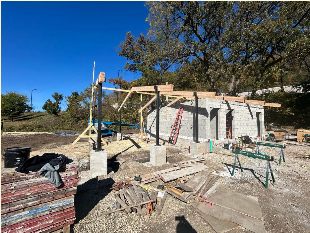
Framing the shelter building
