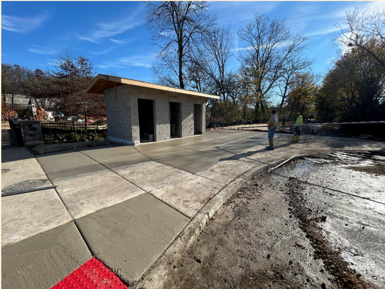
Concrete pour at new restroom facilities
