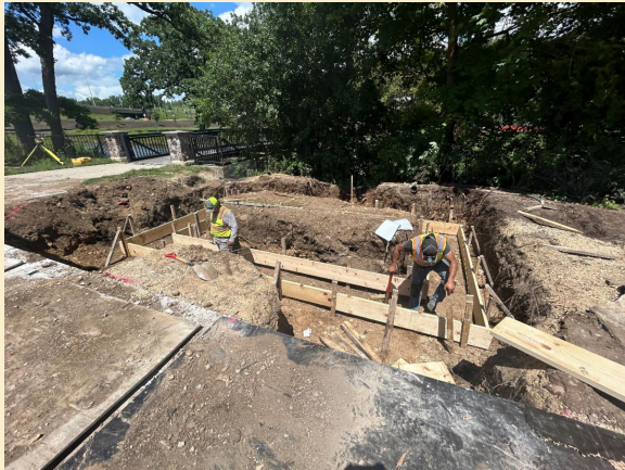
Framing for new restroom facilities
