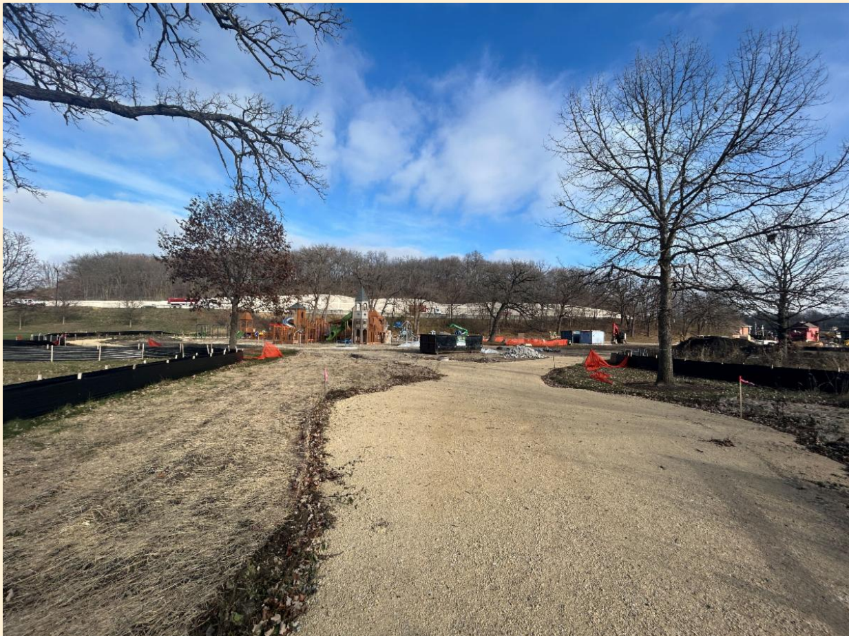
Multi-use path in progress
