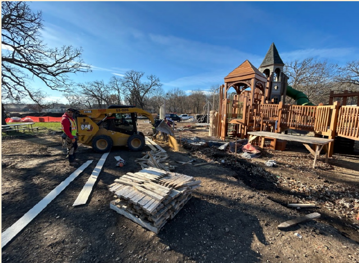
Preparing concrete for the curb and gutter along the playground
