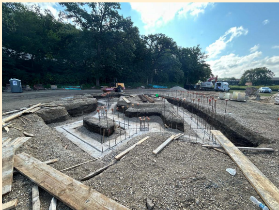
The new bandshell's foundation
