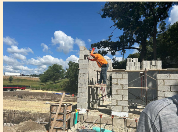
Masonry for the shelter building
