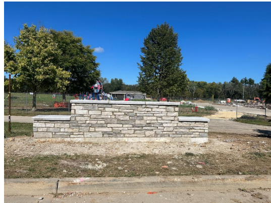
Signage foundation installation
