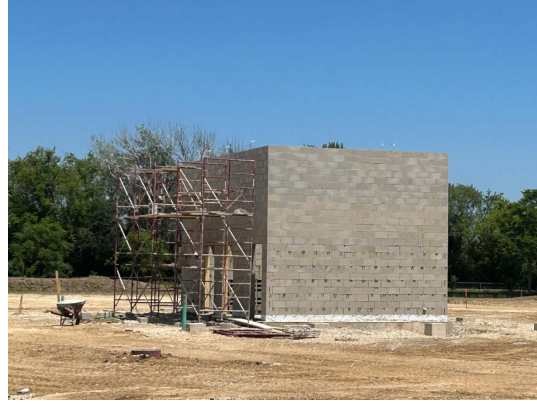
CMU wall installation
